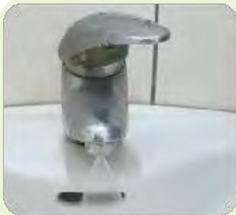
Replacement of water-saving equipment (Installation of aerators)
