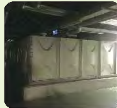
Installation of a water recycling system (Modular water tank recycling system)
