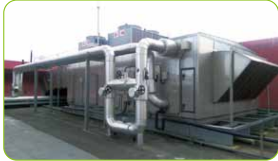
AC system improvements (Installation of a Make-up Air Unit to reduce chiller unit load)
