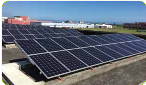
Renewable energy improvements (Installation of solar panels)
