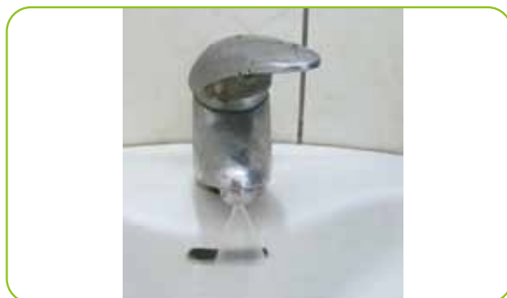
Replacement of water-saving equipment (Installation of aerators)
