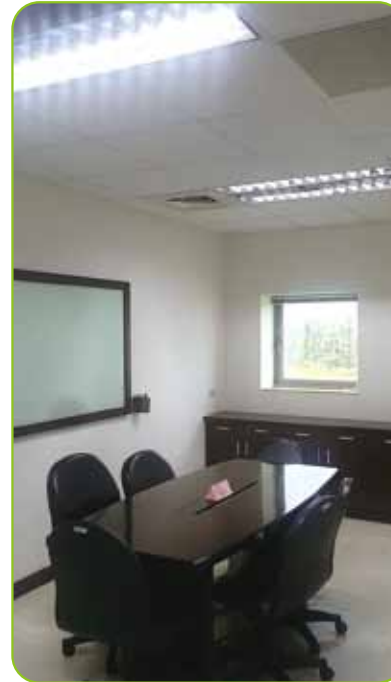
Lighting equipment improvements (Installation of LED lighting devices)
