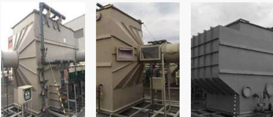
Yilan Plant 3 Addition of washing tower
