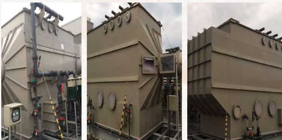
▲ Yilan Branch Plant 3 adds a washing tower
