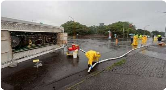
▲ The Containment Team carried out drainage channel containment operations.
