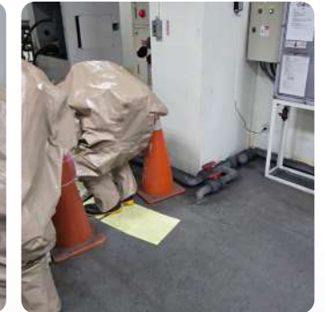
4. The Emergency Rescue Team enters the hot zone: (1) Operate the equipment to stop the acid discharge and contain the leak (2) Place absorbent pads and booms around the leak. (3) Once no residual liquid remains at the leakage site, place the used absorbent pads and booms into hazardous waste disposal bags.
