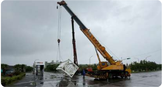
▲ The Tank Transfer Team carried out lifting operations.
